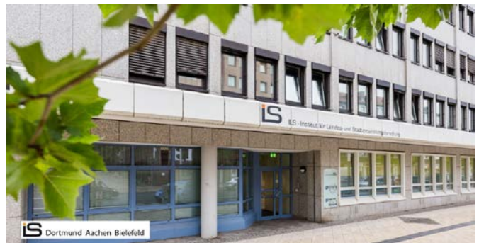
사진 1. The front of ILS building in Dortmund
